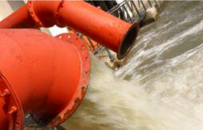
Costs for building and operating water utilities are escalating.
